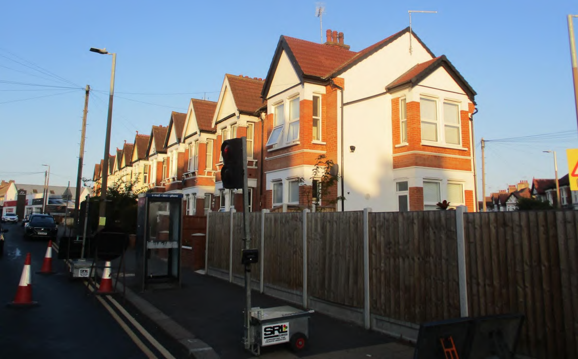
Street Scene looking West
